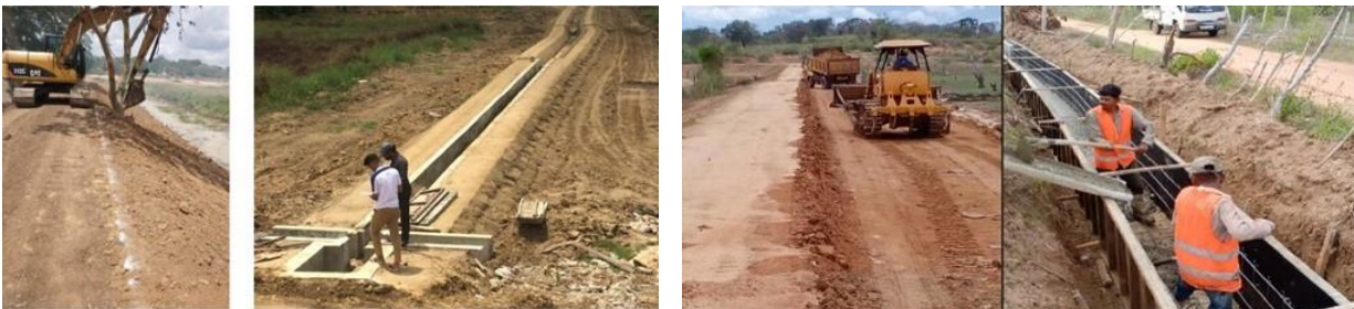
Pic13: Tank and Down Stream rehabilitations
