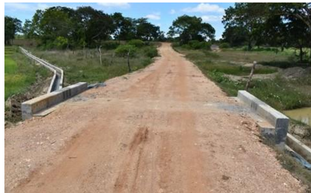
Pic 12: Rehabilitated agri-road
