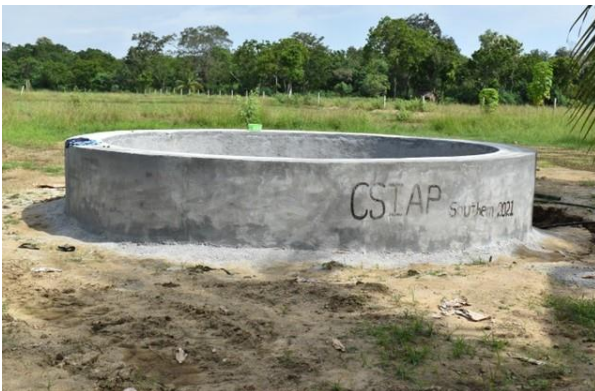
Pic 11: Rehabilitated agro-well
